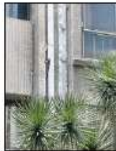
Base station blended into building facade
