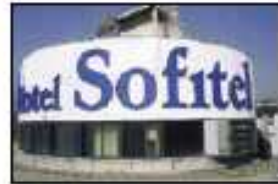
Base station blended into building facade
