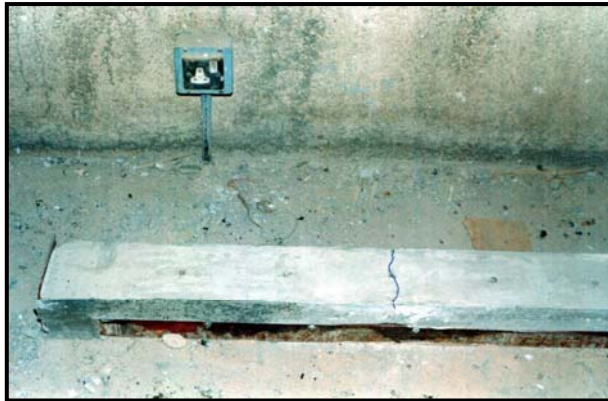
Plate (4.1) : The Crack Location in Specimen (LM 3 )
