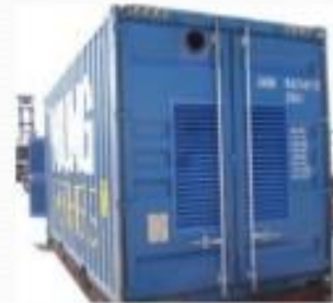
Portable, backup, and stationary generators
