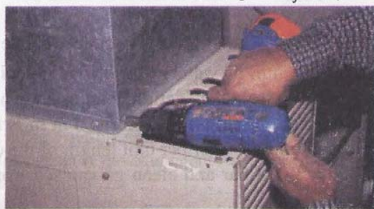
Fastening duct using a portable electric drill and sheet metal screws.
