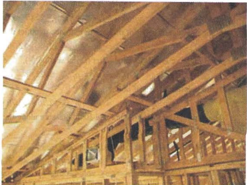
Heating and air - conditioning ducts.
